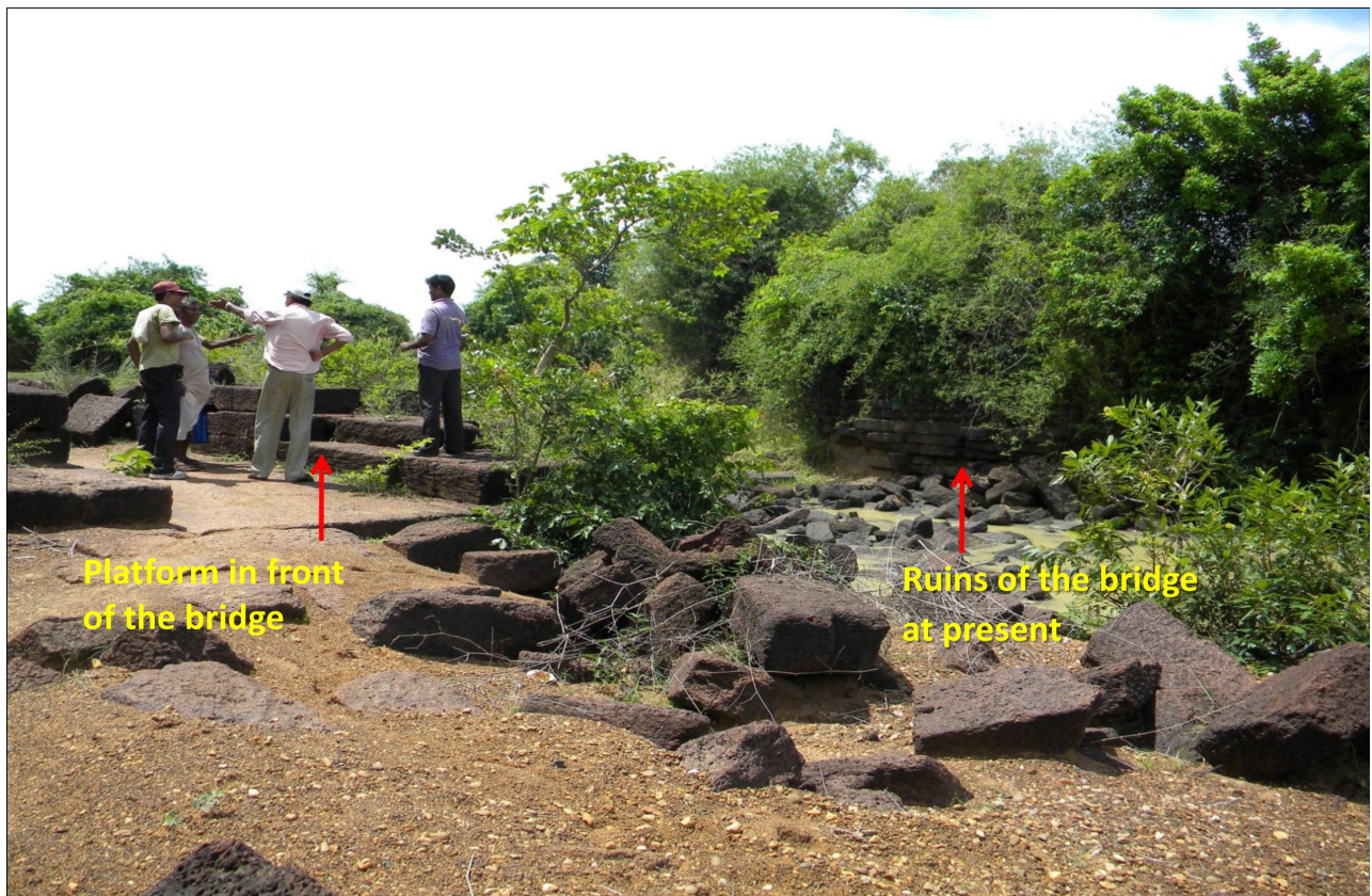
Fig. 11: Remains of Dum Dumi Bridge and Platform
